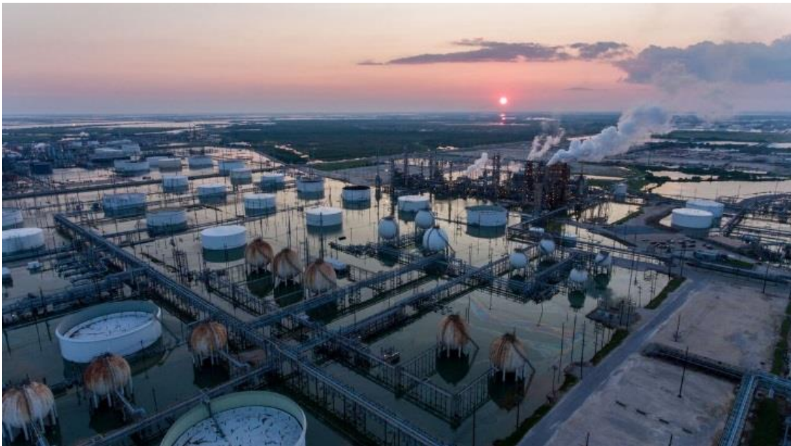
Refinery at Port Arthur 05. Sep. 2017 after Hurricane Harvey: Foto Alexander John Glustrom
